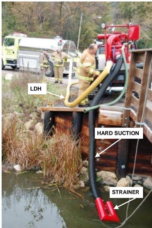
At left, shown is the hard suction (non-collapsible black hose) attached to the red strainer floating on the water, which keeps the suction near the surface (where the water is cleanest). The drafting rig then pumps water through the (yellow) large diameter hose (LDH) to fill the tank of the shuttle (water tender) rig.
