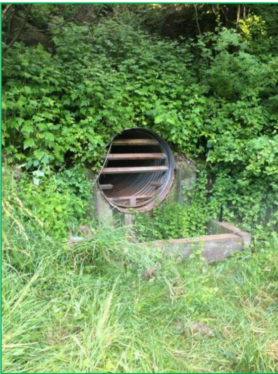
The main ventilation shaft - an unlikely point where the boys may have entered the Neda Mine, but with lacking any other options at the time, it was the home base for the search. (Photo by Clay Christenson)
